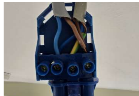
Fault finding and repairs
