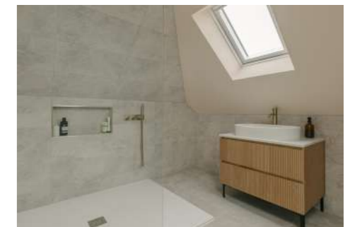
General plumbing services
